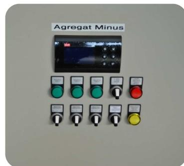
Maintaining a constant suction pressure (by turning on or off individual compressors or control valves on the compressors) allows for fine tuning of the capacity.
